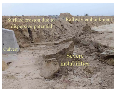
Fig. 2 Severe stability problems occurred at the studied railway embankment after a high rain season during the Spring of 2019
